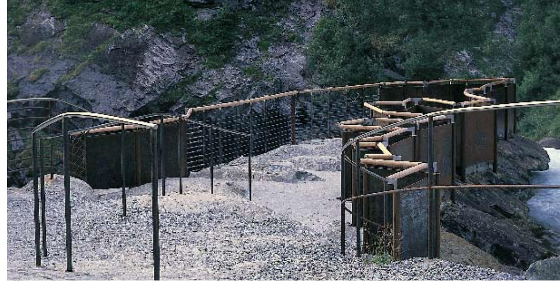
Railings, Videseter falls, Strynefjellet mountain road. Jensen & Skodvin 1997.
